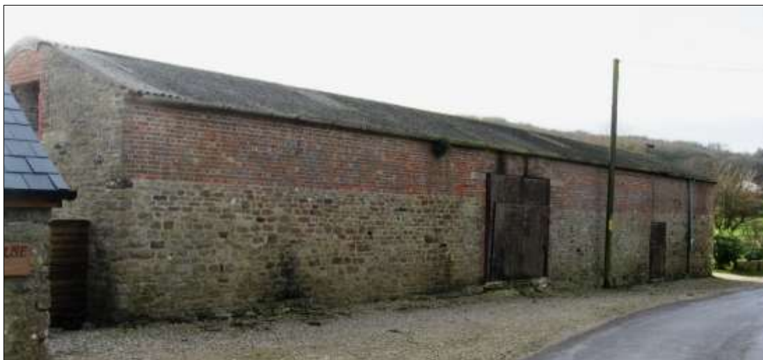
FIG. 11: Stonework. The barn opposite East Creech Farm features a mixture of limestone and heathstone rubble. The walls have been raised in brick. The building was heavily altered during the twentieth century and is compromised by the sheet roof and poorly formed entrance.
