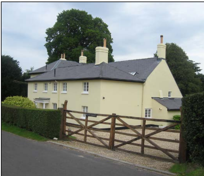
FIG. 31: The Old Vicarage, Higher Street. The roof of this building has recently been re-covered with Welsh slate. The original part of the property is to the rear and can be identified by the steeply pitched roof with catslide – similar to others within the conservation area. Clay tiles are more likely to have covered the original part of the building, though slate would have suited the lower pitches used when remodelled during the nineteenth century.
