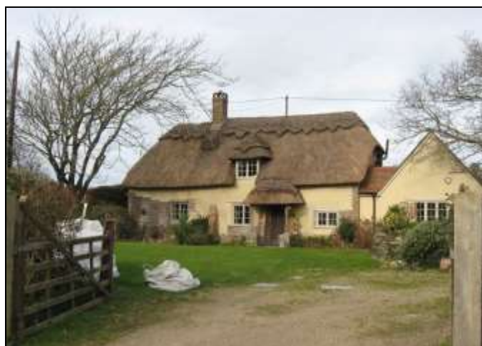
FIG. 13: Wren Cottage. The original part of the structure stands at the centre. The elaborate block ridge is not a traditional feature.
