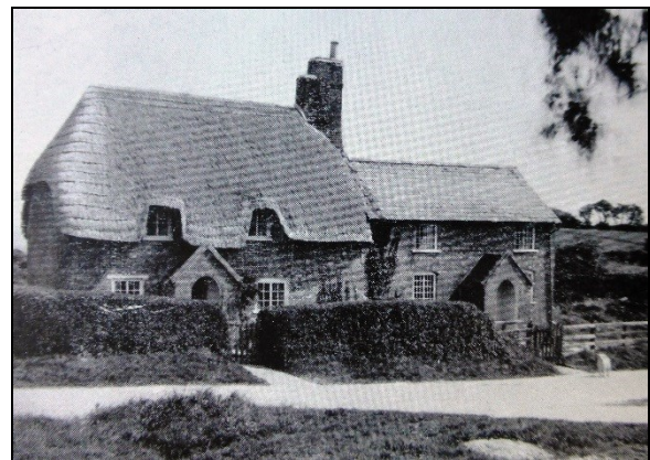
FIG. 2: Rockley Cottage. One of the oldest cottages in the hamlet. Dramatic changes in the appearance of the roof have arisen from replacement of the historic covering as seen by comparing a modern view with one included in the RCHM survey of 1970. The block ridge is a modern feature not typical of the local tradition.
