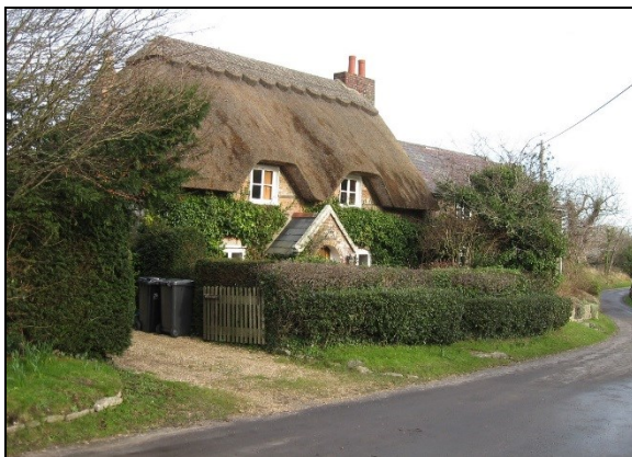
FIG. 2: Rockley Cottage. One of the oldest cottages in the hamlet. Dramatic changes in the appearance of the roof have arisen from replacement of the historic covering as seen by comparing a modern view with one included in the RCHM survey of 1970. The block ridge is a modern feature not typical of the local tradition.
