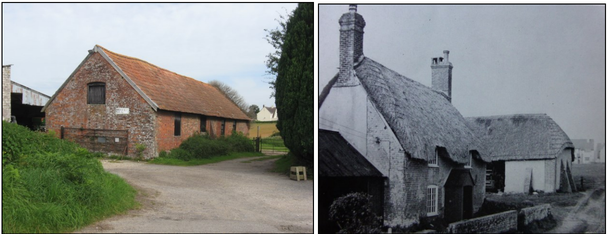
FIG. 8: Eighteenth century farmhouse and barn. Photo (right) taken from the 1970 RCHM survey – see FIG. 6 for position shown on a map. Note modern Council houses on New Road in the background. The thatched buildings were subsequently demolished though a few related buildings (left) remain in use by Sellar's Farm.
