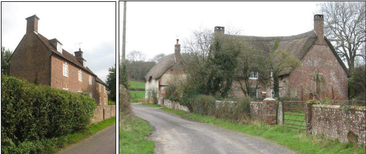
FIG. 21: Architectural variation. Left: Stickland’s Farmhouse, the original part of which features a bold symmetrical frontage with high quality brickwork and detailing. Right: Paddock Cottage and No. 36 West Morden (‘Wayside’), two vernacular structures showing possible variation in historic status.
