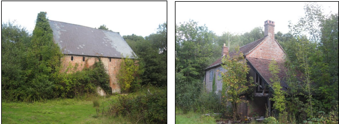
FIG. 14: Morden Mill and Farmhouse. Derelict listed buildings, albeit the farmhouse was inhabited until recently. Note the attached timber framed and clad outbuilding – a common feature of Morden Estate properties around the conservation area. Maps reproduced with the permission of the National Library of Scotland.
