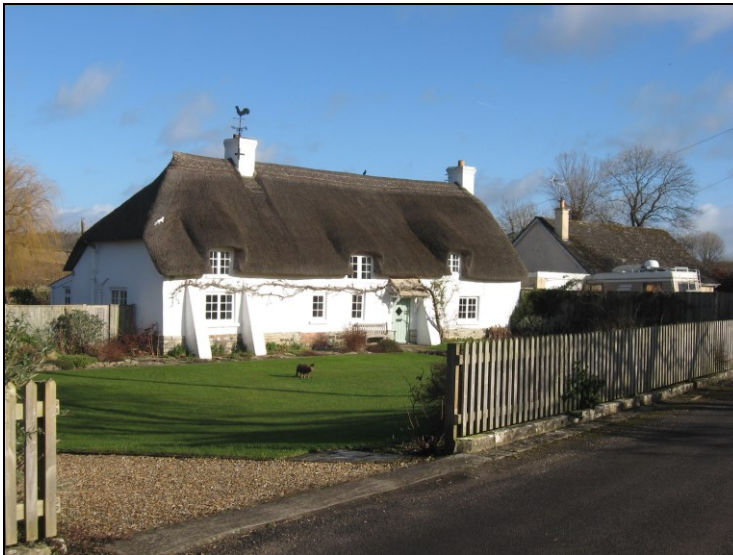
FIG. 4: Cruck Cottage, Briantspuddle. The oldest domestic property in the conservation area, elements of which date to the late fifteenth century.
