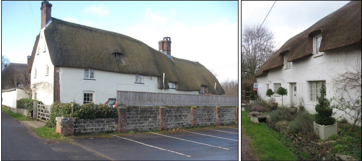
FIG. 5: Seventeenth century. Left: No. 26 Briantspuddle. The oldest section of the former farmhouse stands at 1.5 storeys. Note the deep thatch and exceptional height of the later section of the dwelling. Right: Piper's Cottage, Throop.
