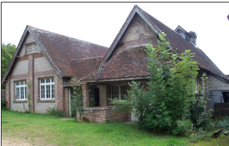
FIG. 13: Dairy building at Tonerspudde Farm. Shown prior to conversion. Typical block and brick construction, unusually domestic in character.
