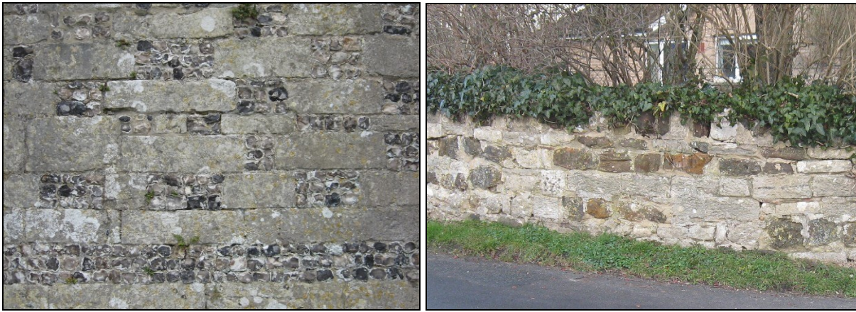
FIG. 19: Stone. Left: Panels of knapped flint used to create a chequered pattern with blocks of limestone at the parish church in Affpuddle. Right: heathstone and limestone rubble in the wall now forming a boundary of Barbaru, Briantspuddle.
