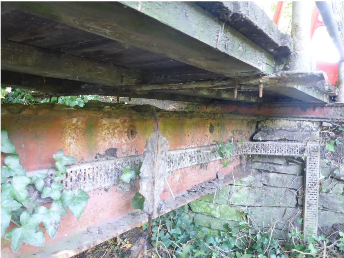
10. Corroded Traverse Beam
