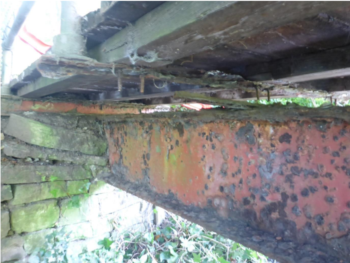
10. Corroded Traverse Beam
