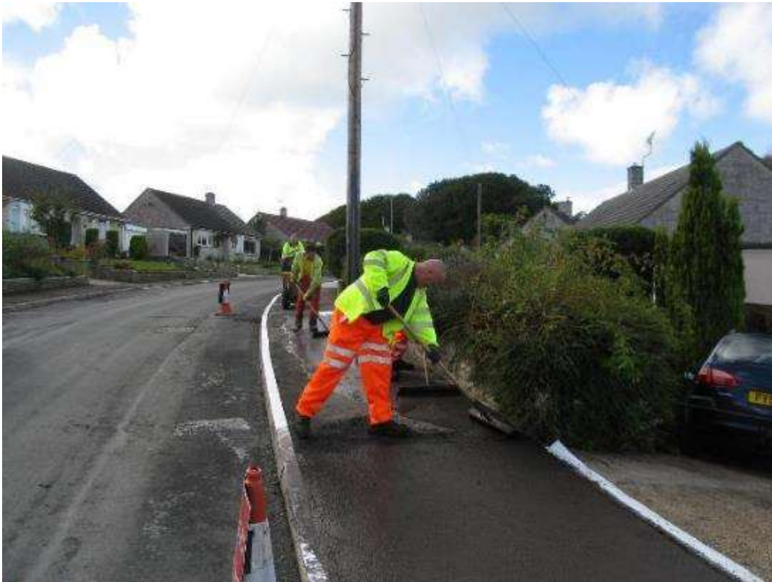
Image Footway slurry seal
