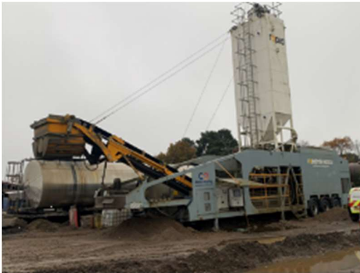
Allasso CBGM Mixing Plant— Ex-situ structural repairs
