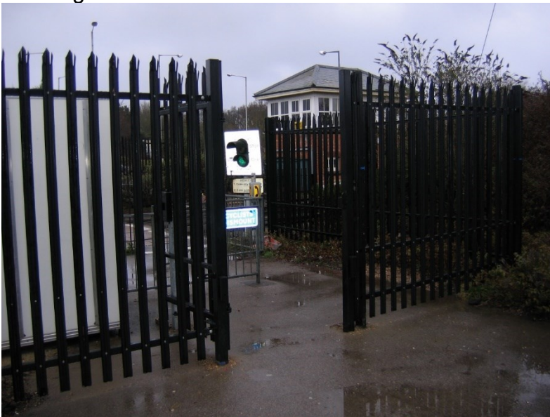
Figure A7. Miniature Stop Lights (MSLs) and external gates controlled by a level crossing attendant
