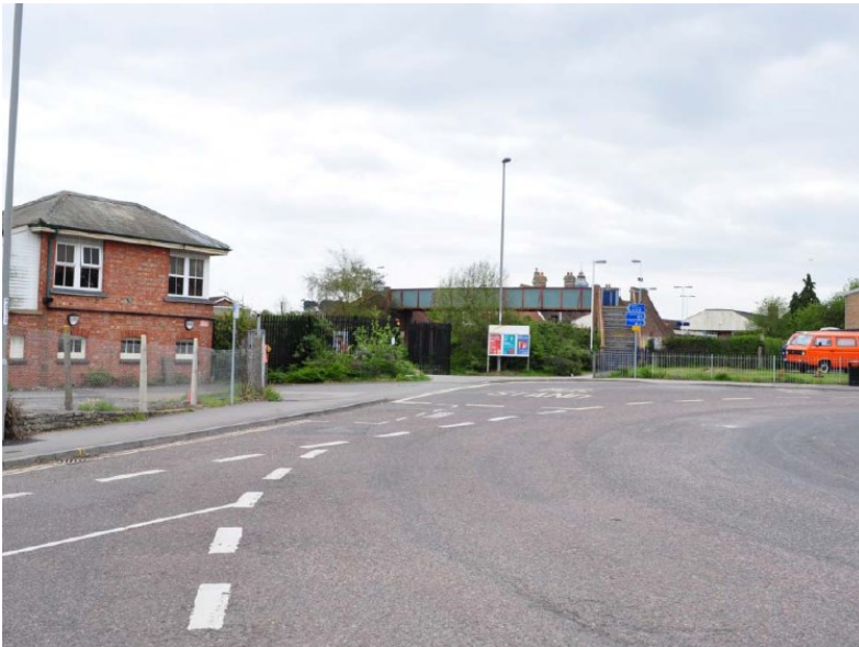
Figure A2. View south from Sandford Road - Bere Road Roundabout showing the location of the pedestrian level crossing and footbridge
