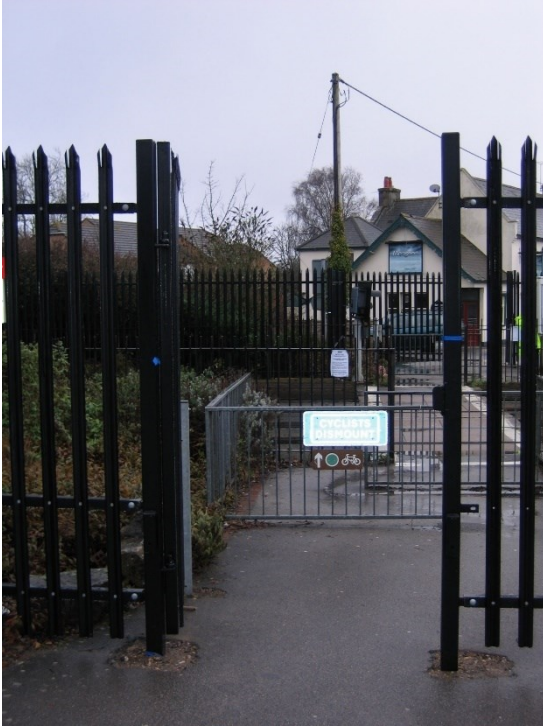
Figure A6. External gates controlled by a level crossing attendant
